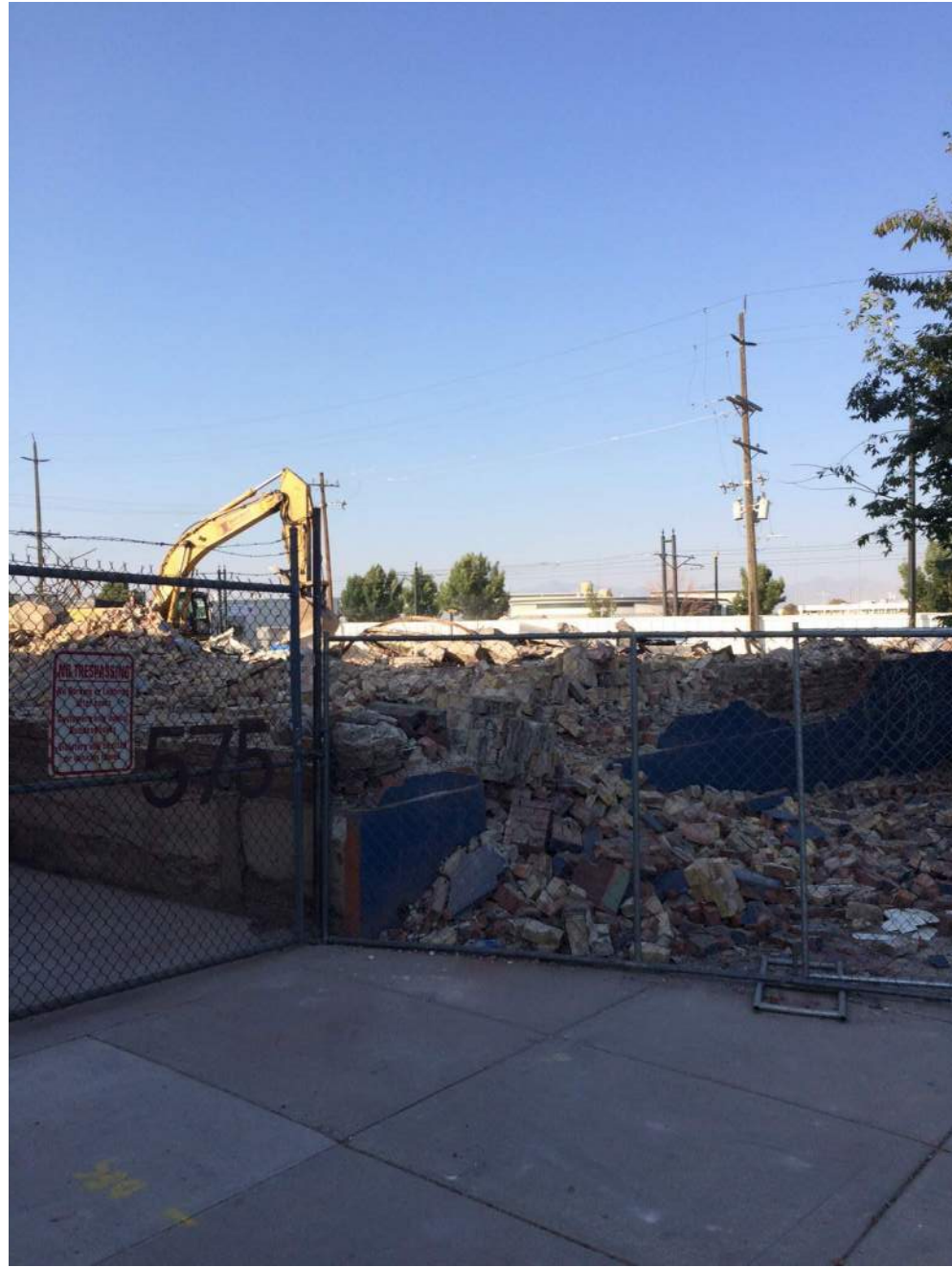
11- ADJACENT CONSTRUCTION PROJECT
